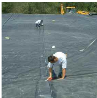
Completing splice detail
