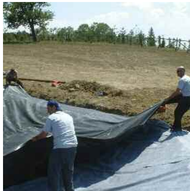
Laying PondGard into trench
