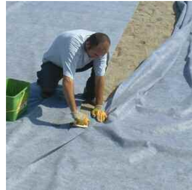
Tacking geotextile underlay
