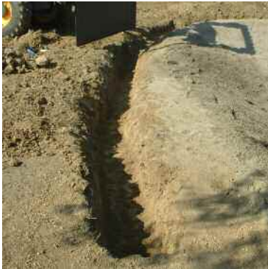
Groundworks anchor trench
