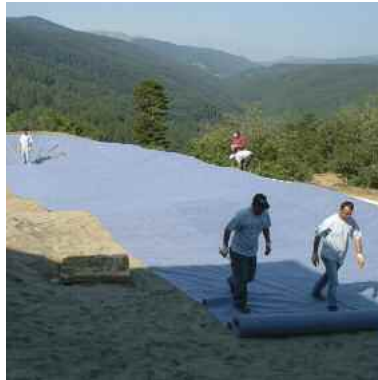
Laying geotextile underlay
