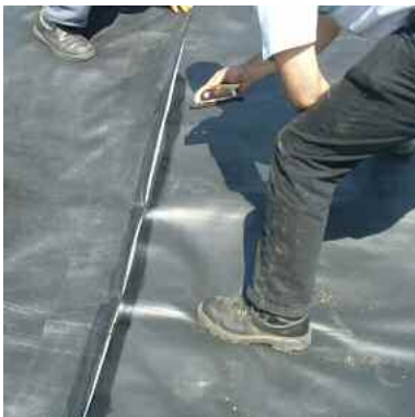
Tacking the splice
