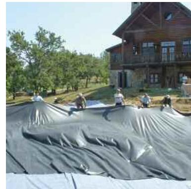
Positioning PondGard sheets
