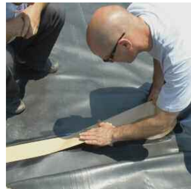
Installing splice tape
