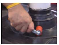
**Step 11**- Using a hand roller; roll the pipe boot flange to insure adhesion to the PondGard panel.
