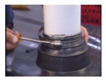
**Step 12**- Attach and tighten the stainless steel clamp to the pipe boot rib that grips the pipe.
