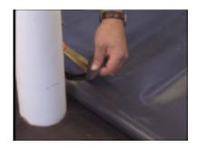
**Step 1**- Cut a hole in the PondGard panel that is approximately 75% of the outside diameter of the pipe protruding from the substrate.
