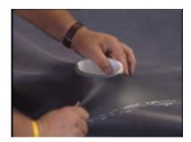
**Step 2**- Then, slide the PondGard panel into place over the base of the pipe.
