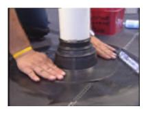
**Step 10**- Smooth the pipe boot flange onto the PondGard panel.
