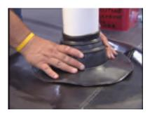
**Step 8**- Slide the pipe boot down over the pipe until the flange of the pipe boot contacts the pre-primed PondGard panel.
