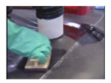
**Step 5**- Using a scrubber pad and holder; apply QuickPrime<sup>™</sup> Plus Primer to a 14.0″ (35.56 cm) diameter area around the pipe. Make sure to extend primer past the adhered pipe boot flange area.
