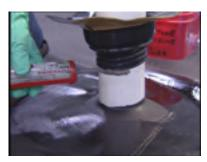
**Step 6**- Place a continuous bead of Water Block Seal at the proper elevation on the boot.
