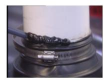
**Step 13**- Apply a continuous bead of Lap Sealant HS or All Purpose Sealant over the top edges and the edges at the base of the boot.
