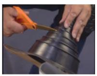
**Step 4**- Using scissors, cut the pipe boot at the vertical rib that is just smaller than the pipe's outside diameter.
