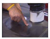
**Step 7**- Test the primer flash-off by touching the primed area with your finger and pushing forward at an angle. The primer should not string as your finger is moved up and away.
